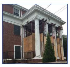
and columns are in critical condition, requiring the installation of scaffolding to provide temporary support in December 2016.
